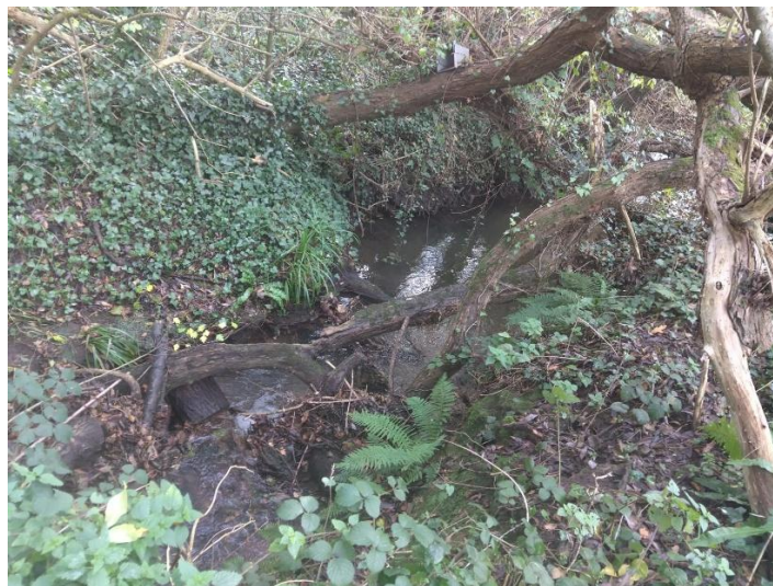
BH03 Minor Woody Material
