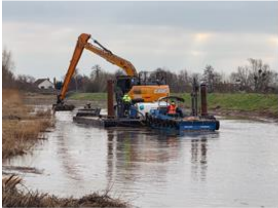
SRA funded dredging of the River Parrett near Moorland, January 2025 (above)
